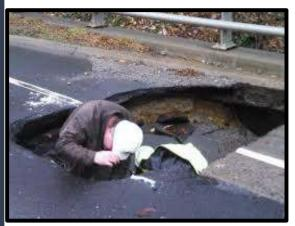
**Consideration Factors:** Engineering and emergency repair crews were quickly on site to determine a plan of action. The erosion was more significant than the 5' x 10' opening, as voids now existed under all lanes of traffic. Repair of the decking was the easy part. Repairing the buried drainage system would not have been as simple.
